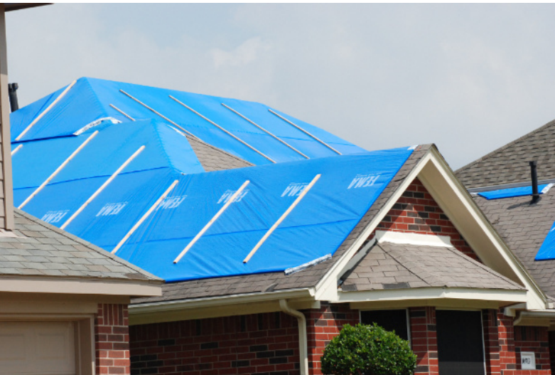
A tarp protects a damaged roof — and the house underneath it — following a hurricane. (Credit: U.S. Army Corps of Engineers.)
